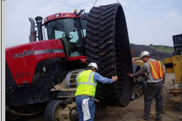
Using a boom truck to remove track
